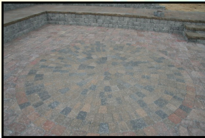
Closeup of floor
